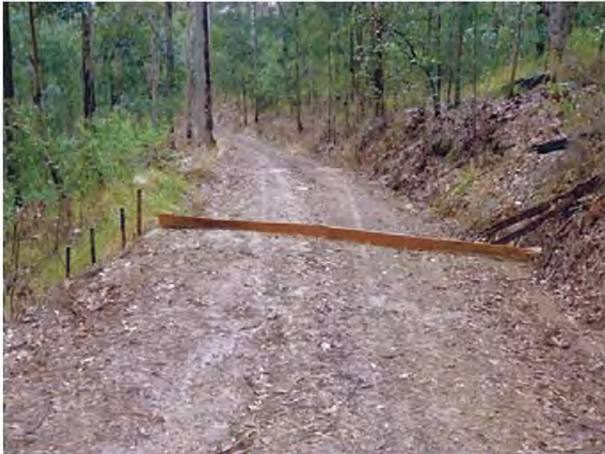
A temporary road drainage structure on a native forest road in coastal NSW (EPA).
